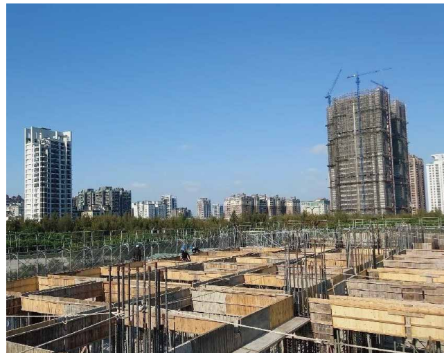
H棟會所-2樓結構施作
